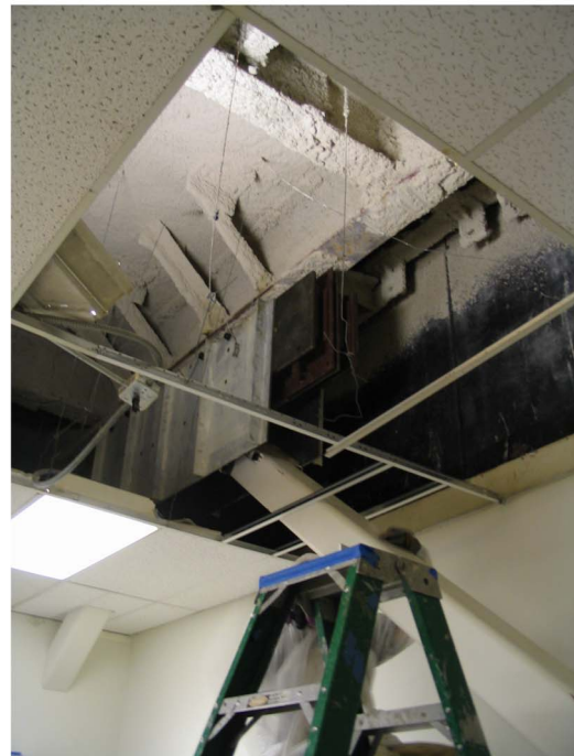
Fig. 12. Photos of: (a) San Mateo County Hall of Justice; (b) view of viscoelastic damper at apex of chevron brace (Photos courtesy of The Crosby Group)
